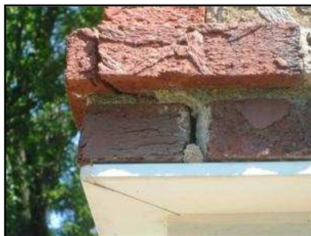
3.0 Picture 4 - SW corner of house.
